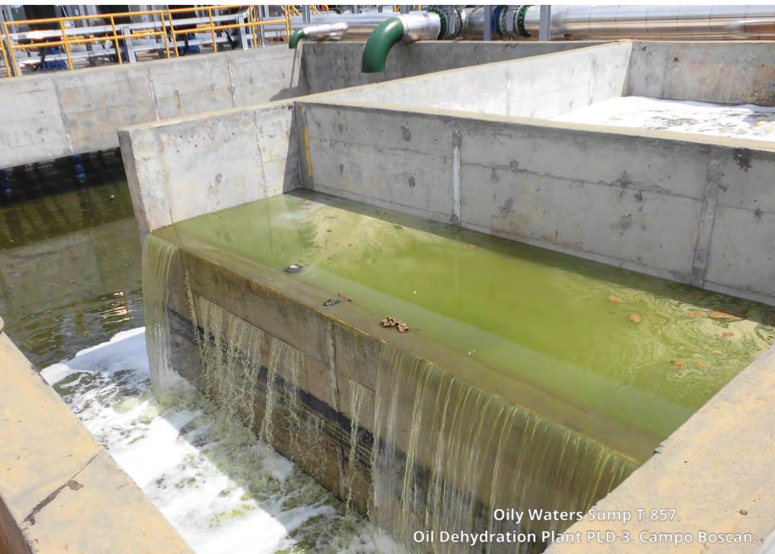
Oily Waters Sump T-857. Oil Dehydration Plant PLD-3. Campo Boscan.
