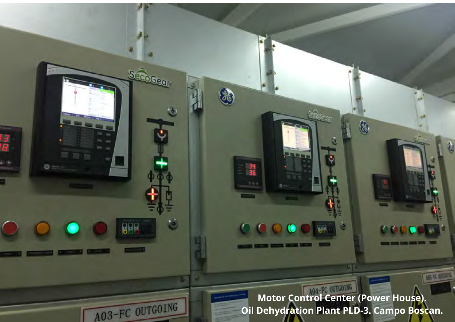
Motor Control Center (Power House). Oil Dehydration Plant PLD-3. Campo Boscan.
